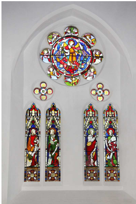
The west window has been repaired and reinstalled. See page 5.
