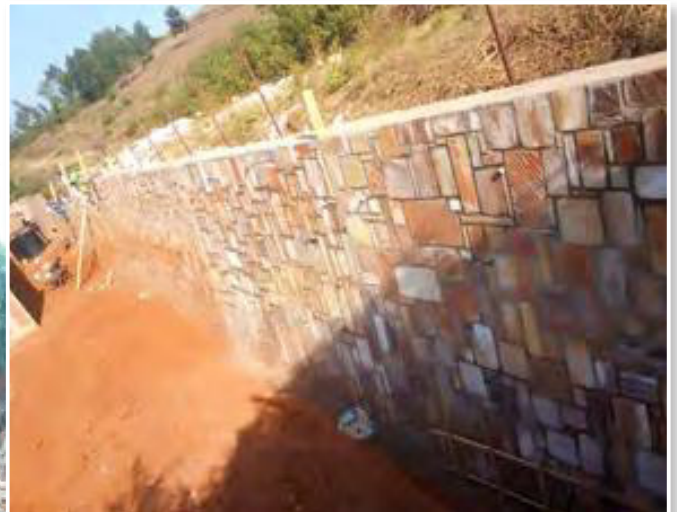
Construction of the stone retaining wall
