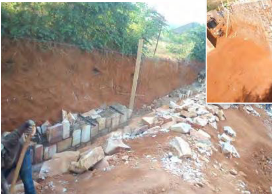
Construction of the stone retaining wall
